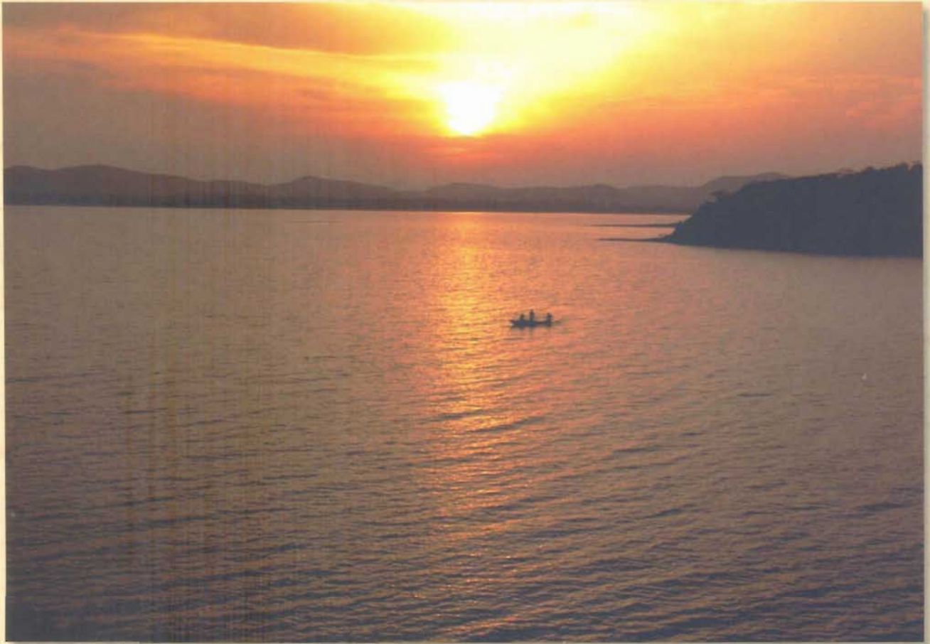
Parakrama Samudra "the sea of Parakrama" built by King Parakramabahu I (1153-86 A.D.) which is the largest irrigation reservoir constructed in ancient Sri Lanka.
