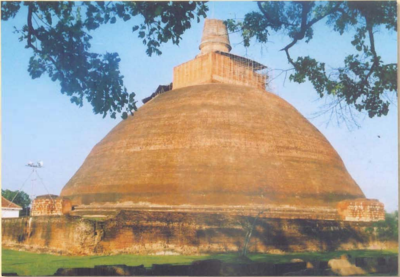
The Jethawana Dagoba, erected by King Mahasena in the fourth century, which is regarded as the tallest brick structure in the world measuring 360 feet in height and consisting of 62 Million ancient bricks. The stupa which is also a UNESCO world heritage site is seen here after renovation.
