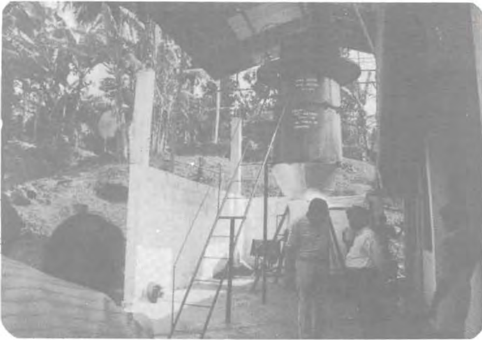
Wood gasifier installed at Morawaka tea factory for drying tea
