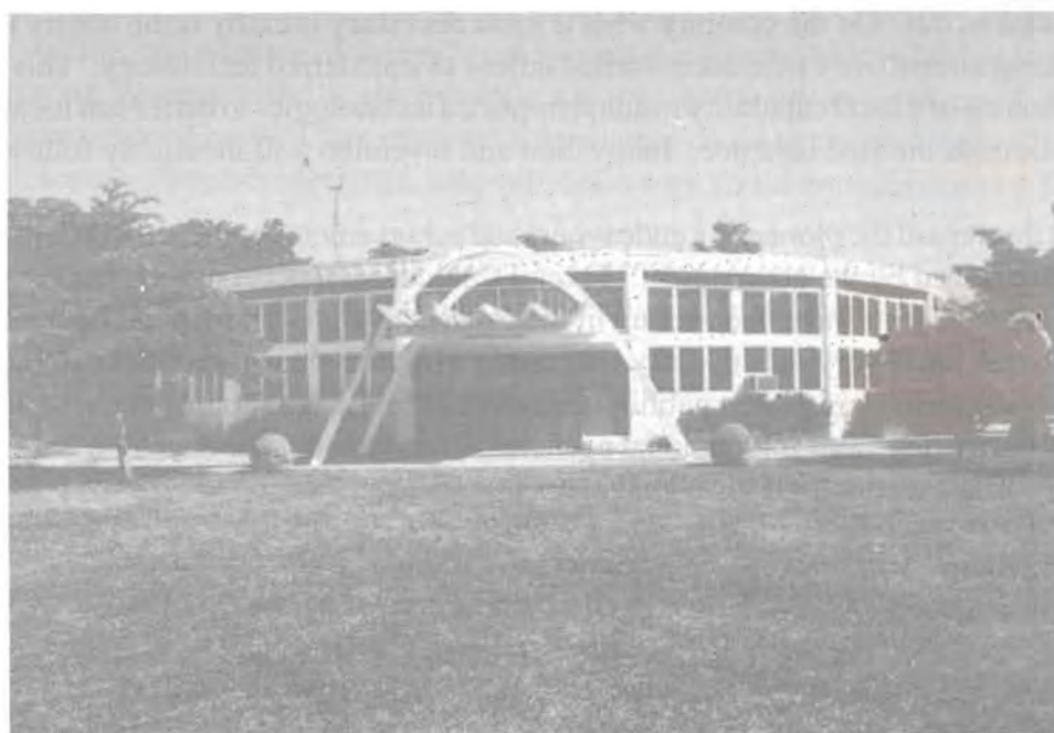
Shell - roof large span public buildings
