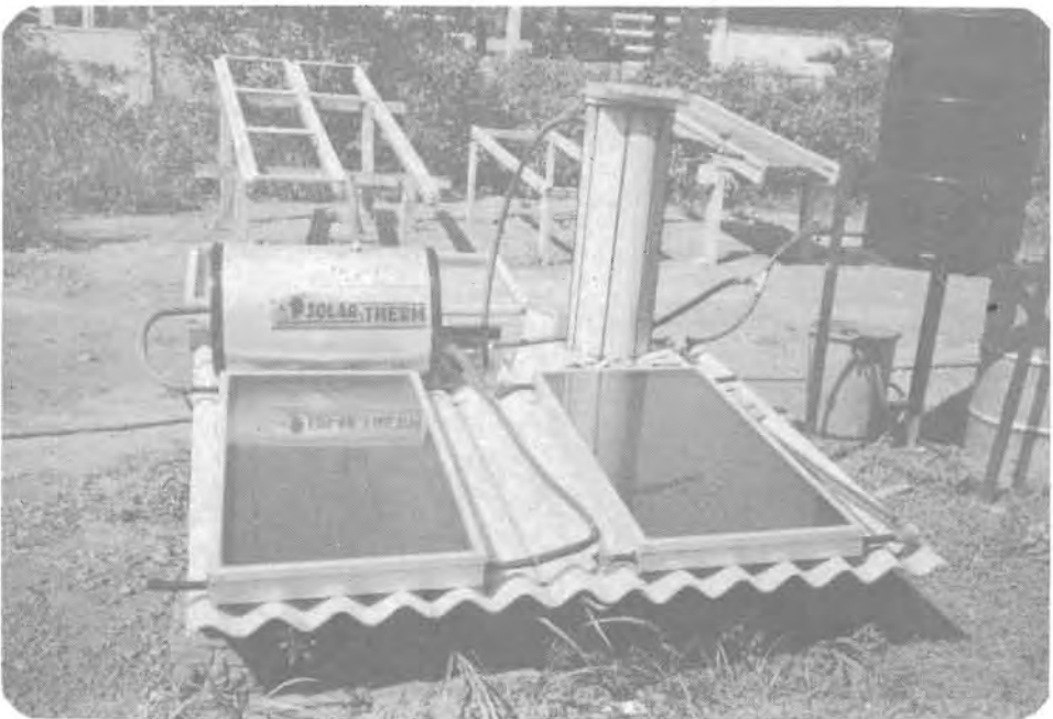
Solar water heaters with horizontal and vertical tanks
