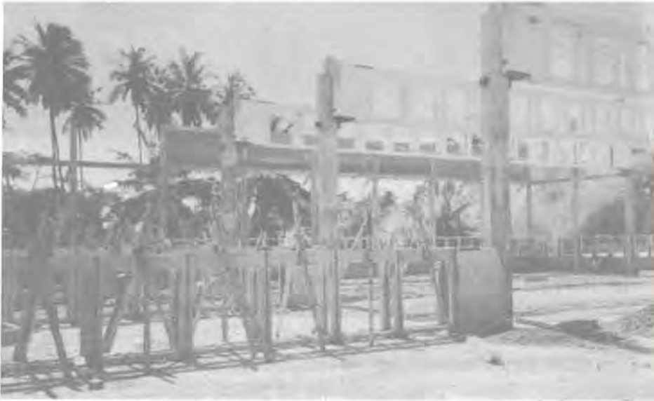
Workshop building under construction
