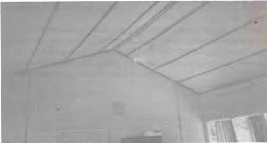
Inside, view of laboratory building showing ceiling
