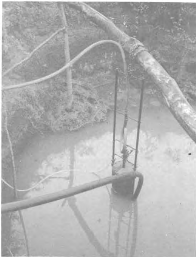
Windmill operated pneumatic water pump installed and in operation
