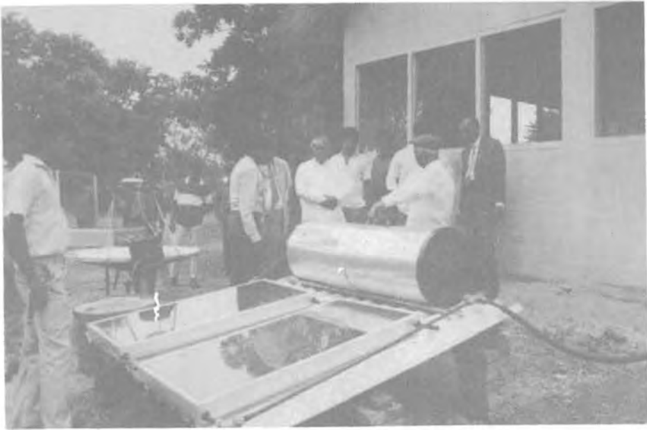
Solar water heater with 30 gallon horizontal tank
