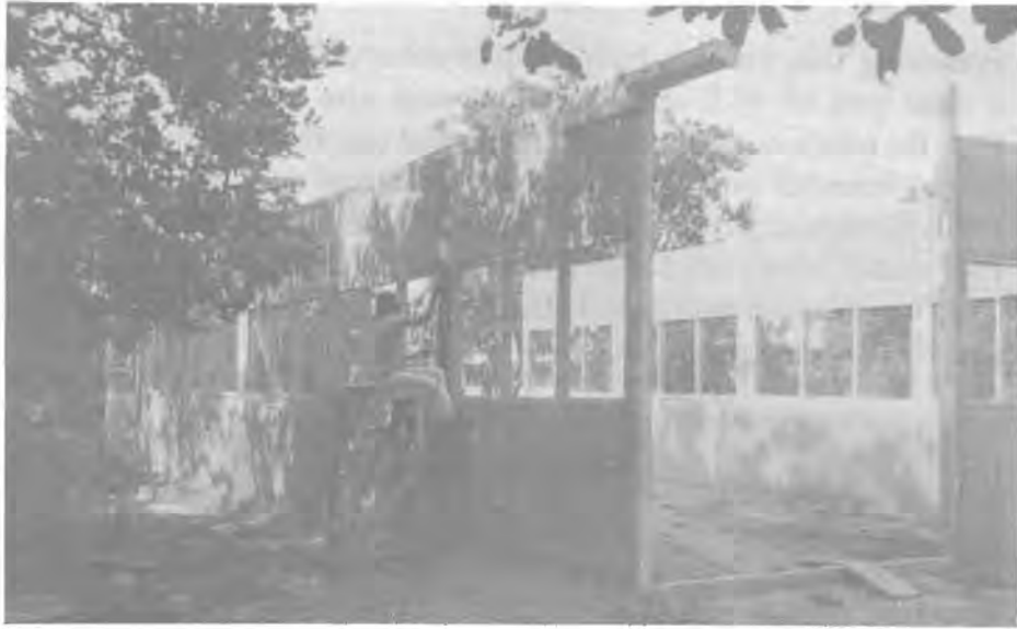
Civil Engineering building under construction
