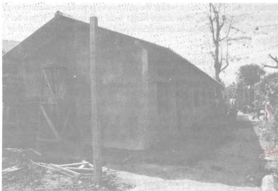
Low - cost house on going construction
