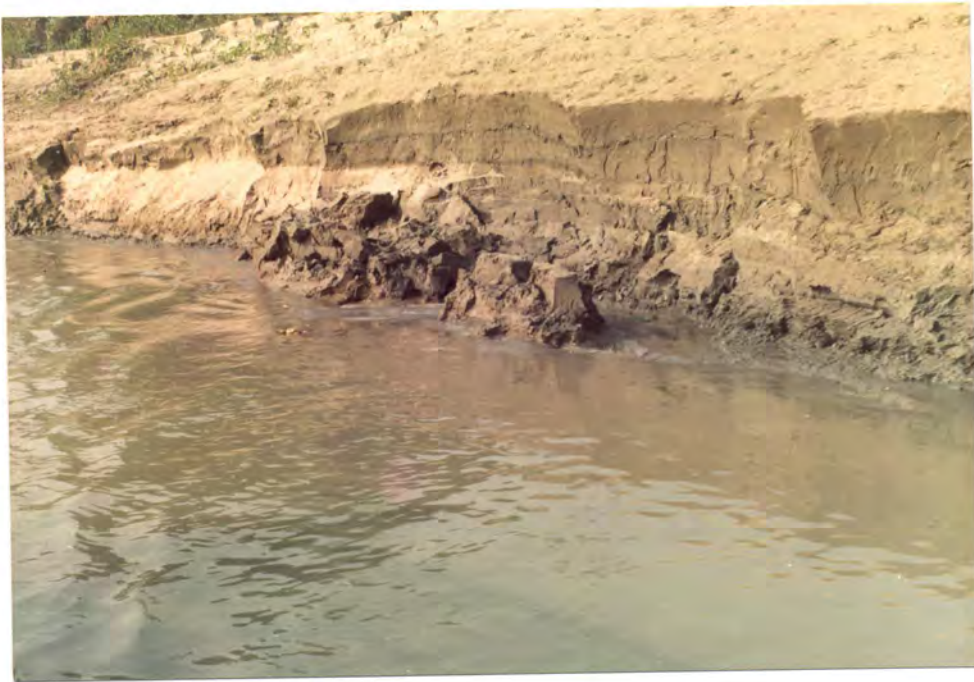
River bank erosion
