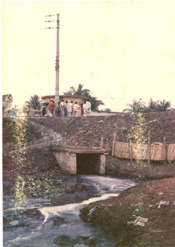
Outfall of sewer being discharged directly without treatment.
