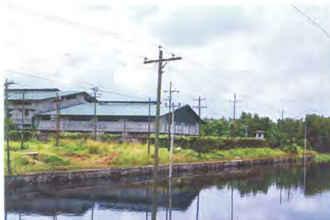
A view of industries, situated on the river banks
