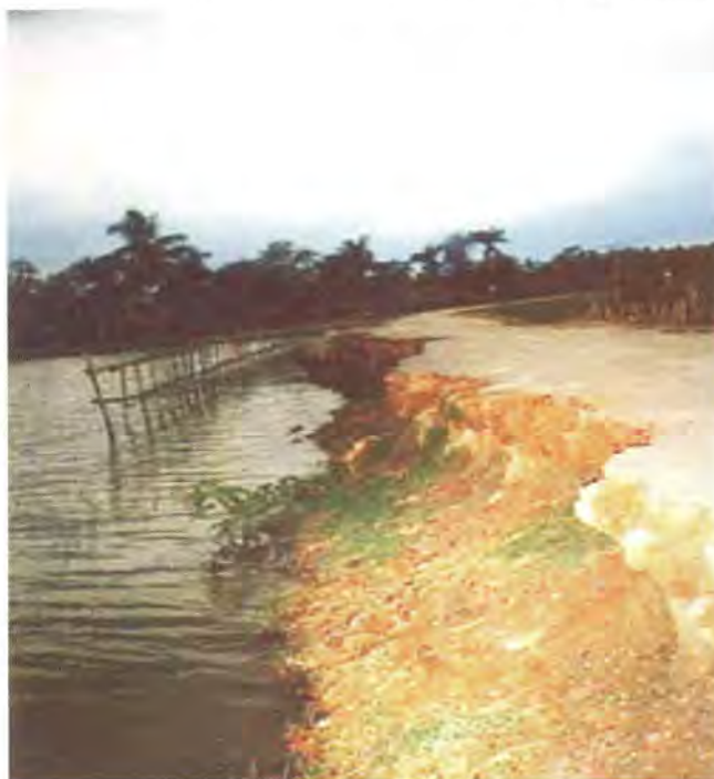
River bank erosion
