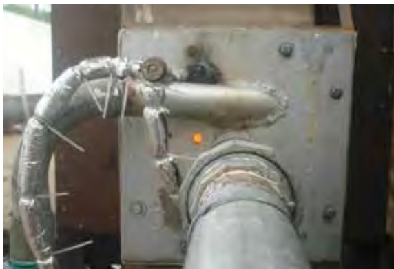
Biochar Plant at Operation
