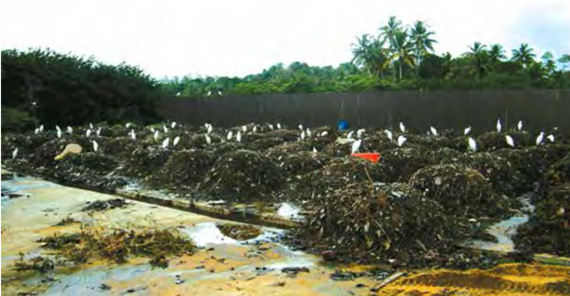
Compost piles at the Weligama Urban Council, one of the pioneer urban councils in the country in composting municipal solid waste. EFL supported the expansion of the Weligama Urban Council composting facility.
