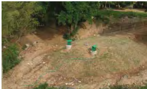
Leachate Treatment Bioreactor
