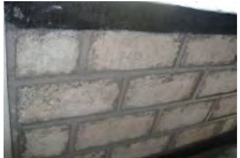
Sludge brick wall
