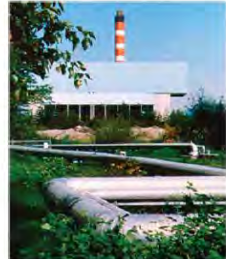
Metro Vancouver's Waste-To-Energy Facility: steam line carries steam to adjacent paper recycling mill and displaces their use of fossil fuels
