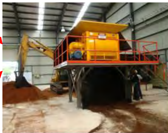
Mixing Saw dust and Sludge in Sludge Mixer
