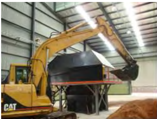
Feeding Saw Dust by Excavator
