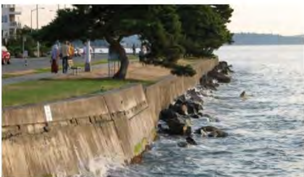
This is a seawall along Harbor Avenue Southwest in the West Seattle neighborhood in Seattle, Washington.
