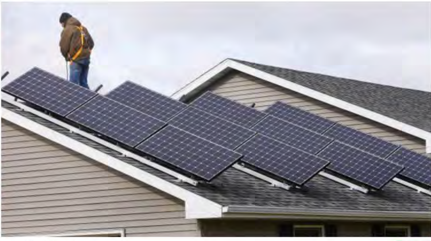
PHOTO BY MIKE DEVRIES An installer with Full Spectrum Solar of Madison installs solar panels at a home near Belleville.
