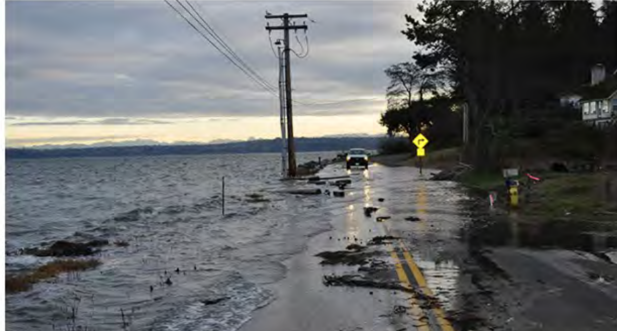
Nuisance flooding in Port Orchard, WA on January 6, 2010.
