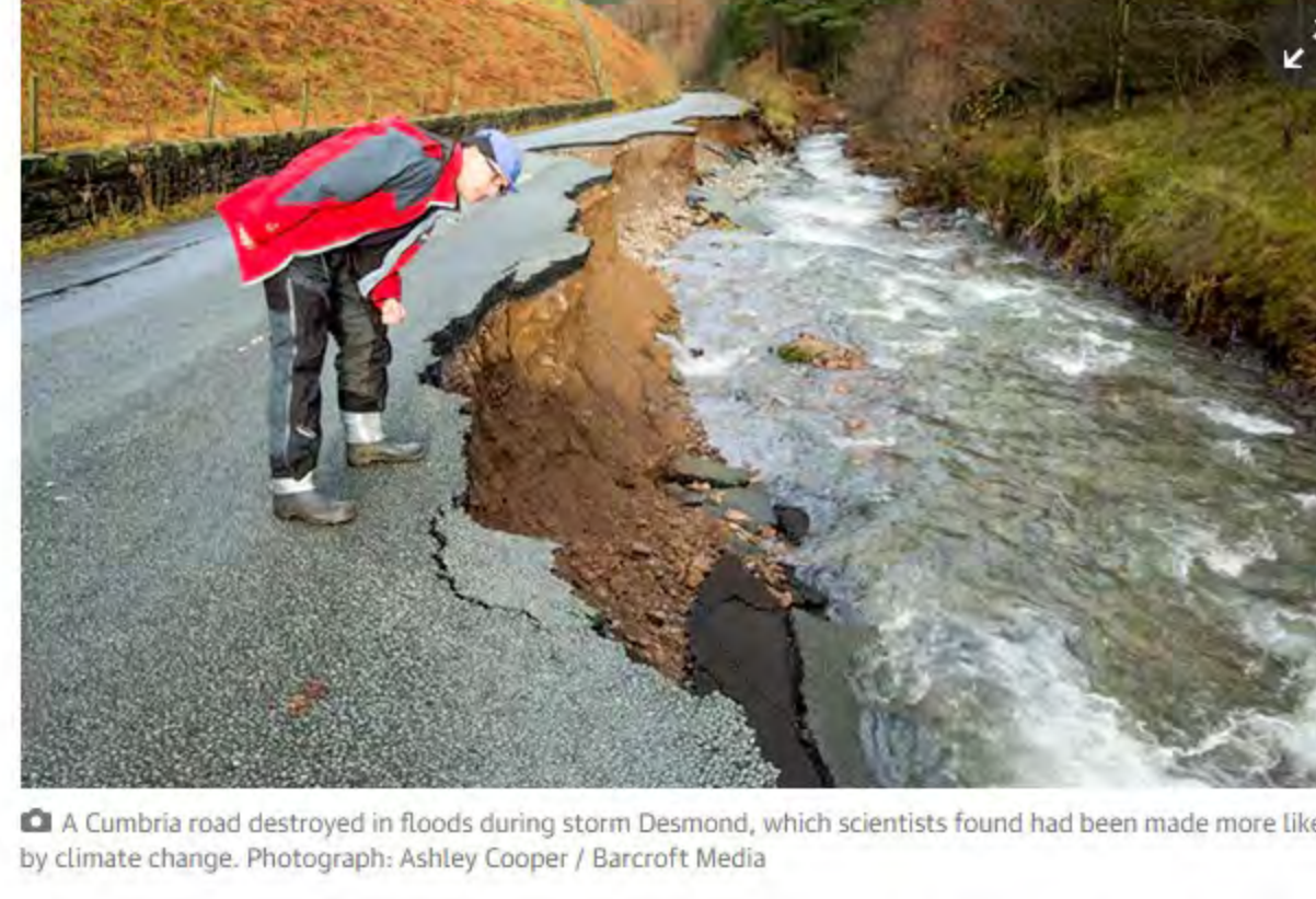
A Cumbria road destroyed in floods during storm Desmond, which scientists found had been made more likely by climate change. Photograph: Ashley Cooper / Barcroft Media
