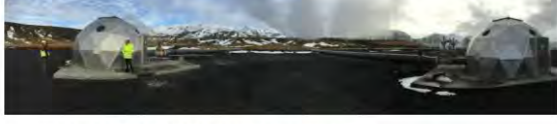
The carbon injection site at the Hellisheidi complex.
