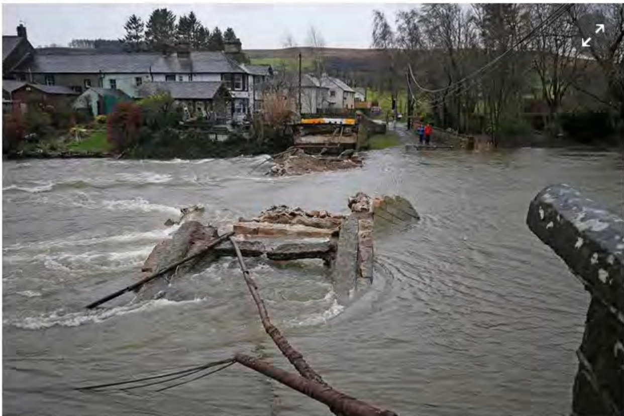
Pooley Bridge in Ullswater, washed away during flooding in Cumbria in December 2015. Photograph: Owen Humphreys/PA
