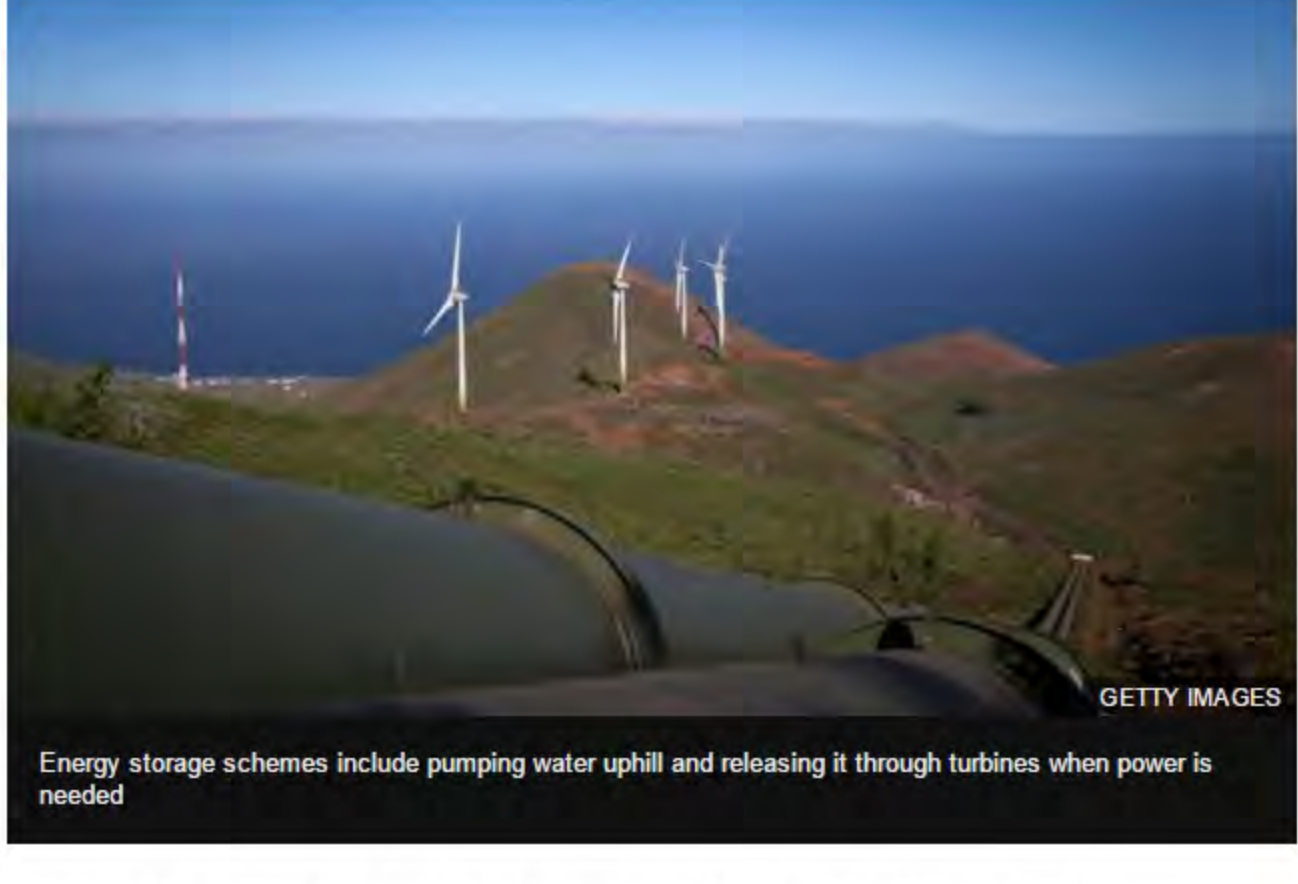
Energy storage schemes include pumping water uphill and releasing it through turbines when power is needed
