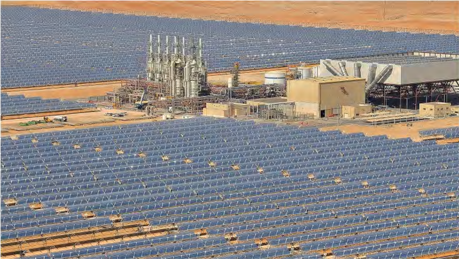
Concentrated solar power plants can store energy for flexible generation (Flickr/Masdar Official)
