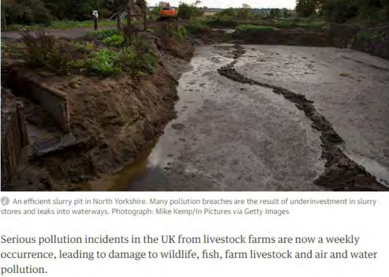
An efficient slurry pit in North Yorkshire. Many pollution breaches are the result of underinvestment in slurry stores and leaks into waterways. Photograph: Mike Kemp/In Pictures via Getty Images
