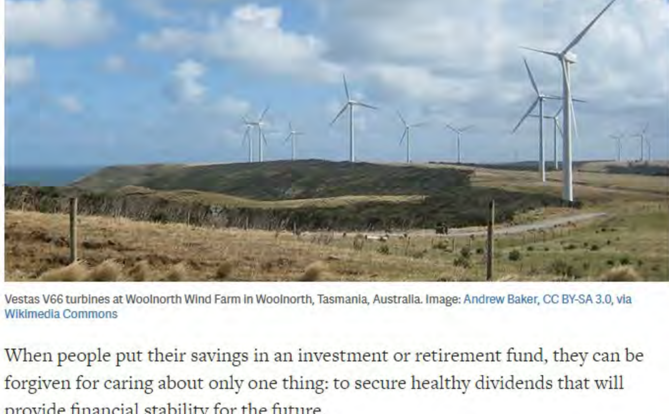
Vestas V66 turbines at Woolnorth Wind Farm in Woolnorth, Tasmania, Australia. Image: Andrew Baker, CC BY-SA 3.0, via Wikimedia Commons
