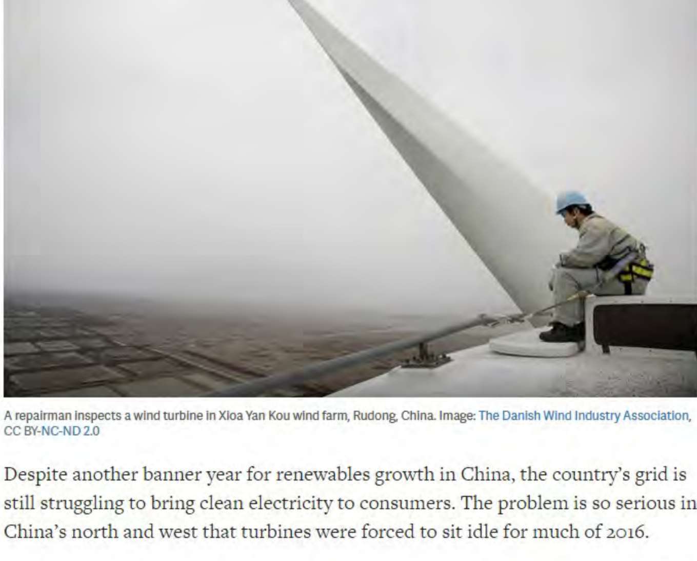
A repairman inspects a wind turbine in Xiaoyan Kou wind farm, Rudong, China. Image: The Danish Wind Industry Association, CC BY-NC-ND 2.0
