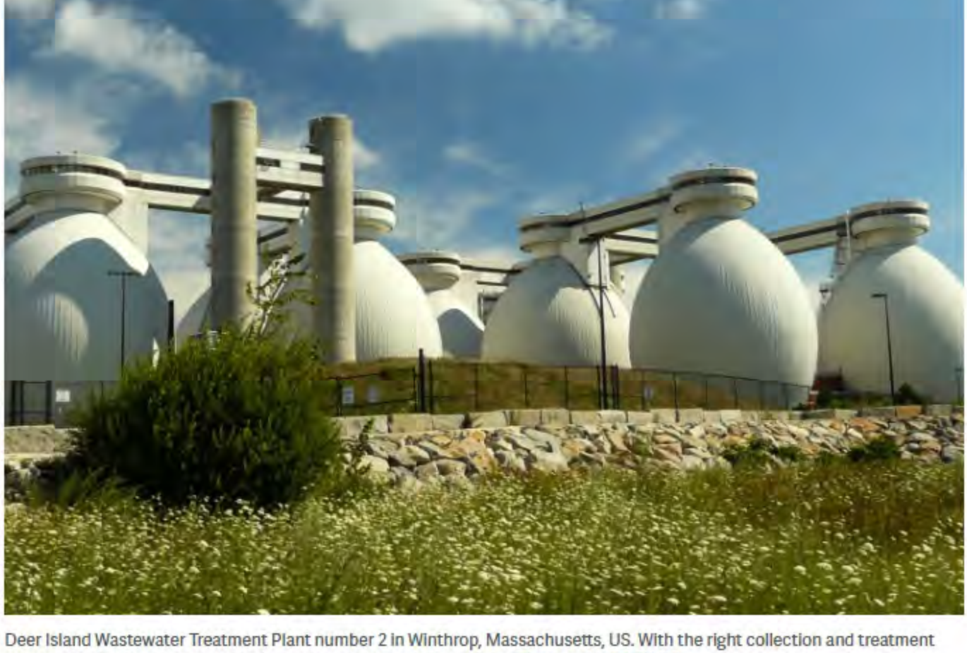
Deer Island Wastewater Treatment Plant number 2 in Wintthrop, Massachusetts, US. With the right collection and treatment systems in place, wastewater can become a resource. Image: Henry Zbyszynski, CC BY 2.0
