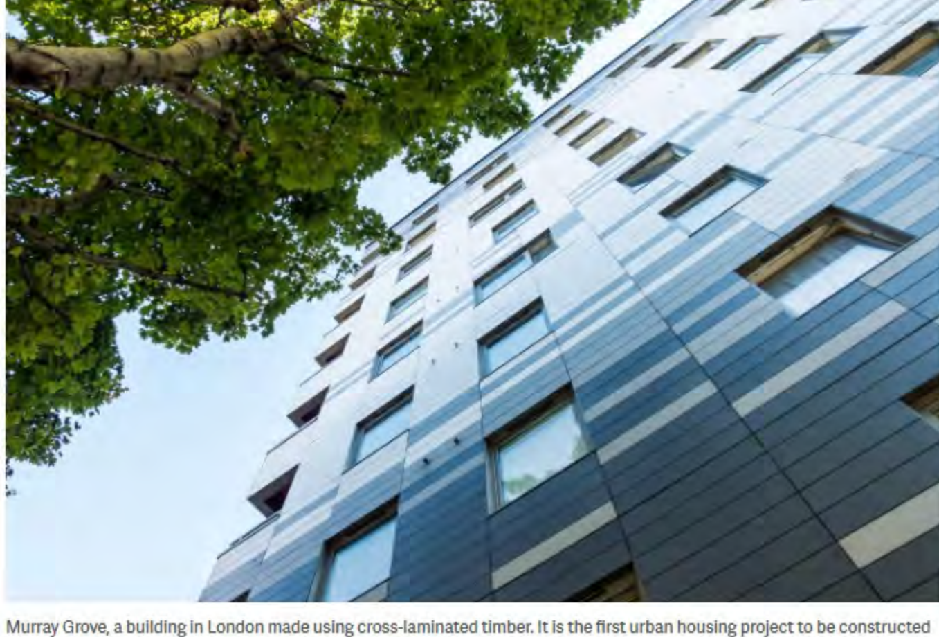
Murray Grove, a building in London made using cross-laminated timber. It is the first urban housing project to be constructed entirely from solid timber. Image: Ben Schuchman, CC BY-NC 2.0
