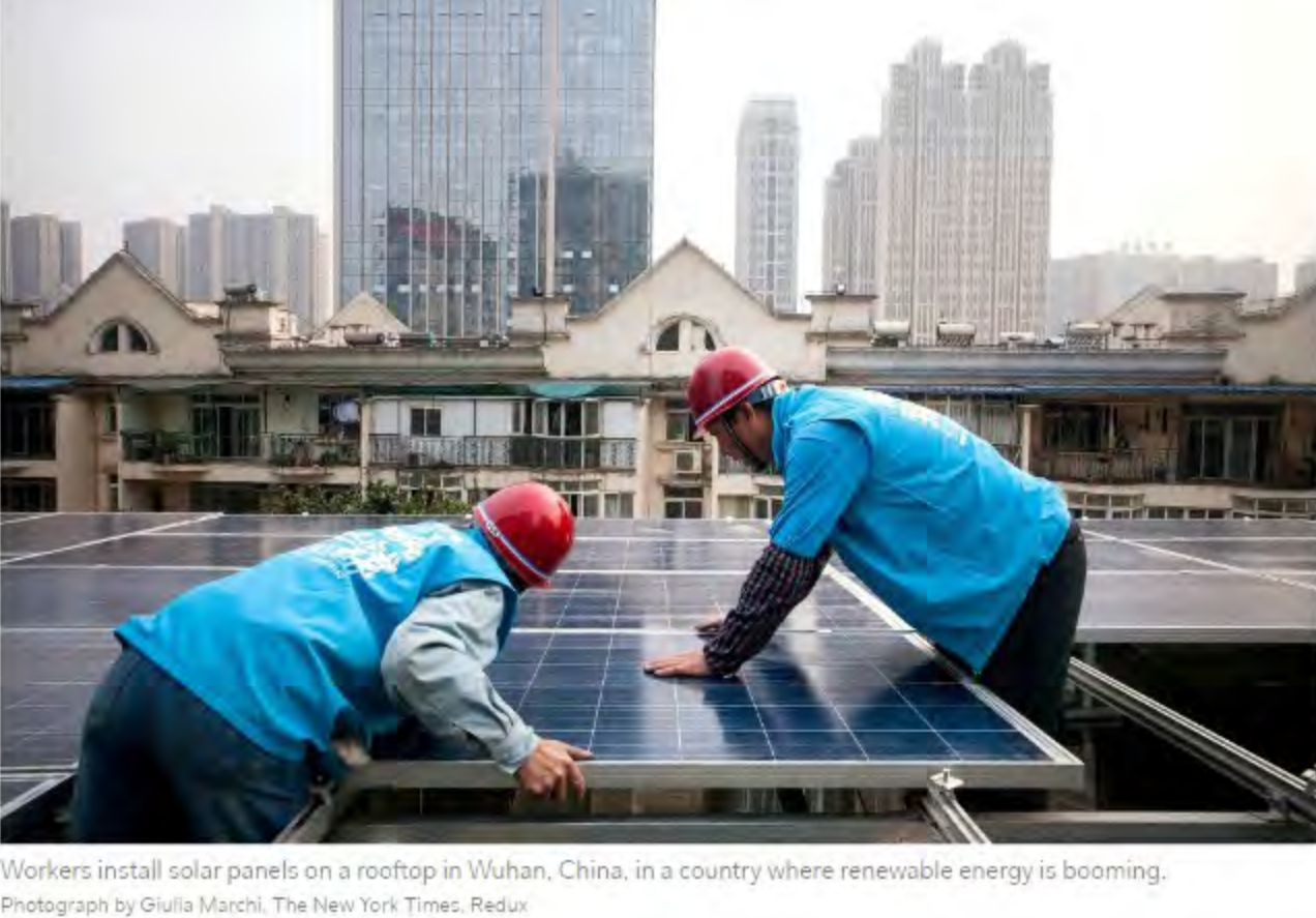
Workers install solar panels on a rooftop in Wuhan, China, in a country where renewable energy is booming. Photograph by Giulia Marchi, The New York Times; Redux
