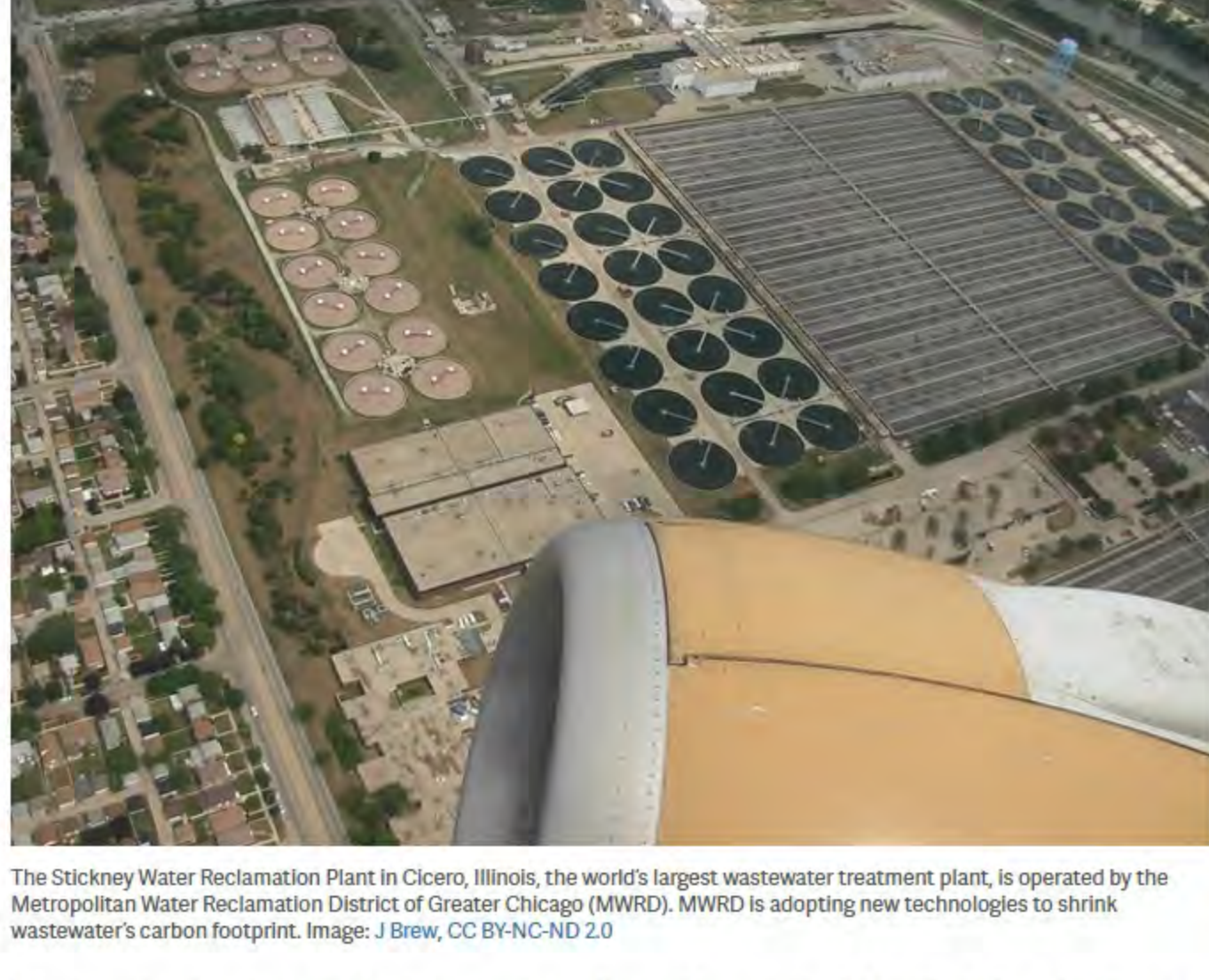
The Stickney Water Reclamation Plant in Cicero, Illinois, the world's largest wastewater treatment plant, is operated by the Metropolitan Water Reclamation District of Greater Chicago (MWRD). MWRD is adopting new technologies to shrink wastewater's carbon footprint. Image: J. Brew, CC BY-NC-ND 2.0
