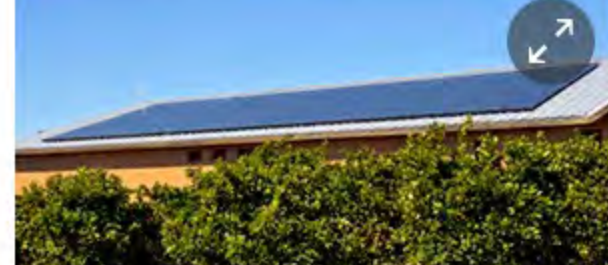
Solar panels on the roof of citrus plant central Florida. The scale of solar power generation in the state lags way behind that in less sun-blessed states. Photograph: Alamy Stock Photo
