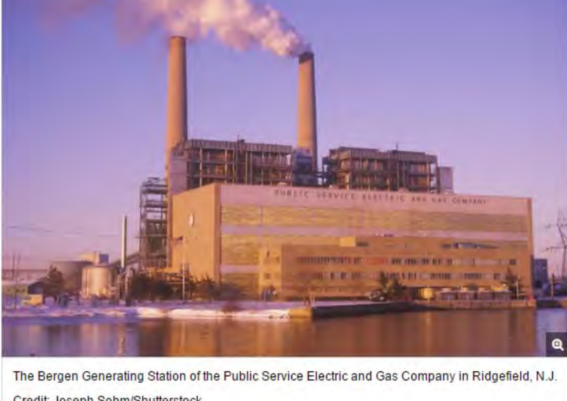
The Bergen Generating Station of the Public Service Electric and Gas Company in Ridgefield, N.J. Credit: Joseph Sohm/Shutterstock
