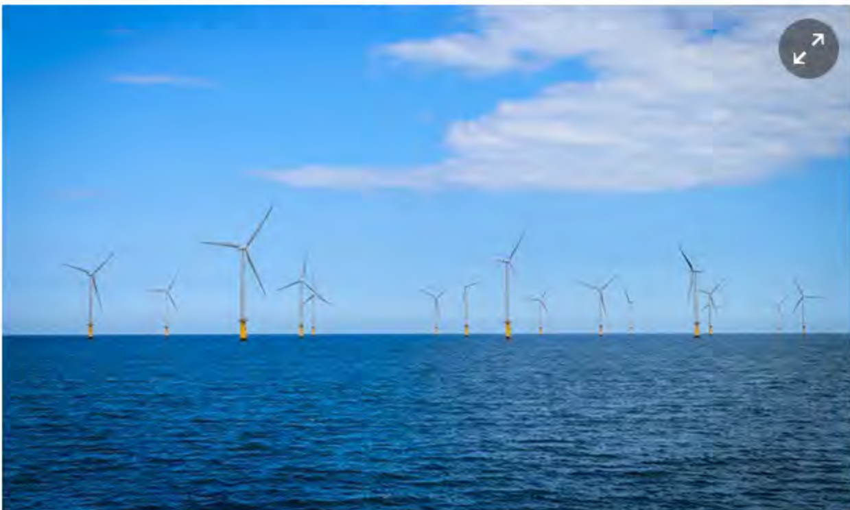
Vattenfall is building Wales' largest windfarm, which is due to come online next year. Photograph: Kapook2981/Getty Images/Stockphoto
