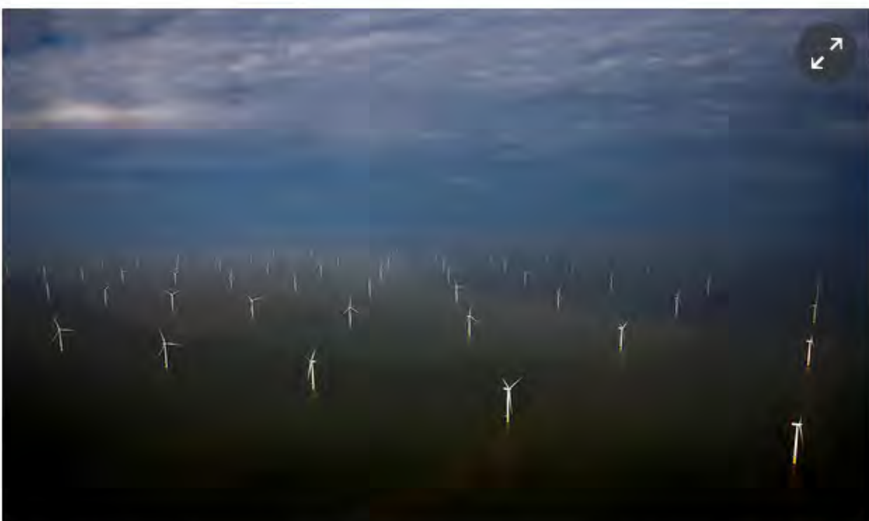
The London Array offshore windfarm. Photograph: Bloomberg/Bloomberg via Getty Images
