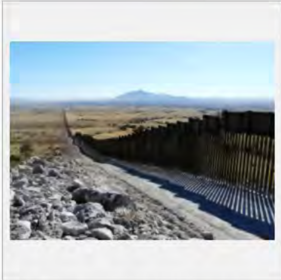
IMAGE: AT THE US-MEXICO BORDER AT THE CORONADO NATIONAL MEMORIAL/ROOSEVELT EASEMENT. THE WALL AND WIDE PATROL ROAD CAUSE HABITAT FRAGMENTATION, THREATENING THE WELL-BEING OF MANY SPECIES. view more >
