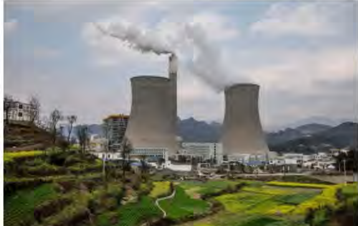
This coal-fired power plant in Guizhou province is one of China's newer ones. The country leads the world in carbon emissions—but also in investments in renewable energy.
