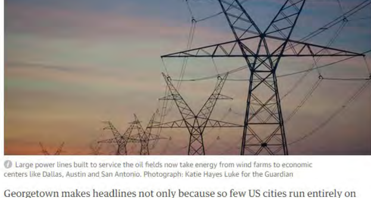
Large power lines built to service the oil fields now take energy from wind farms to economic centers like Dallas, Austin and San Antonio. Photograph: Katie Hayes Luke for the Guardian
